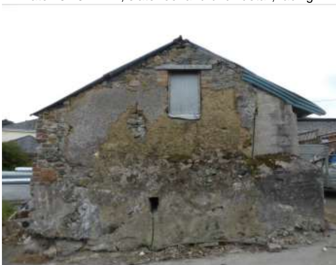
Plate 13.17: BH 3, northern gable showing stone footing,
