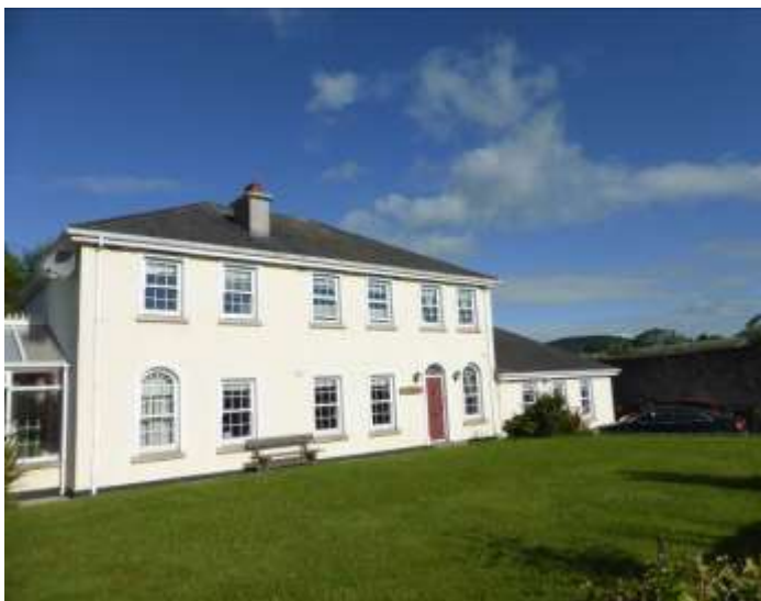
Plate 13.13: Farrankelly House, facing northwest
