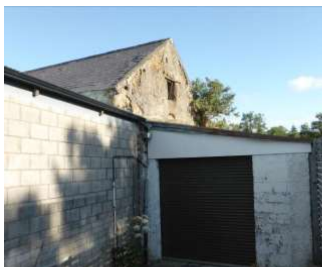
Plate 13.24: BH 5, rebuilt block wall and modern
