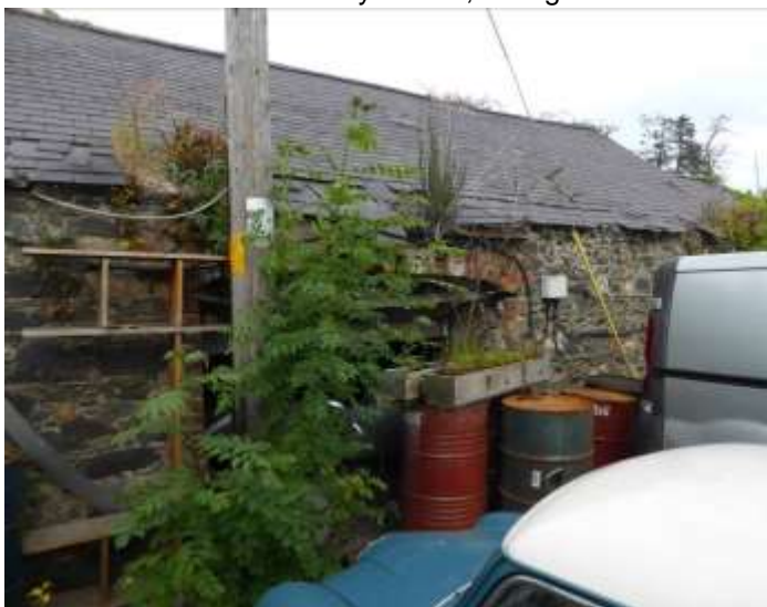
Plate 13.15 BH 1, slate roof and brick detail, facing
