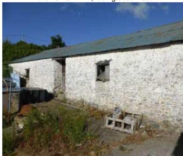
Plate 13.18: Eastern wall of BH 3, rebuilt in stone
