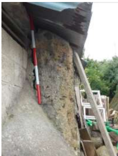
Plate 13.19: BH 3, width of cob wall where western wall
